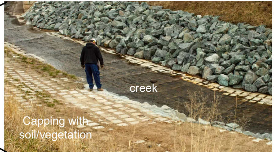
Erosion control system
